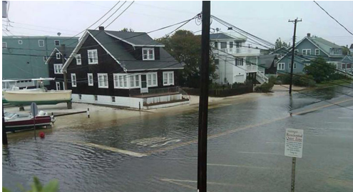
Inland flooding in the streets of this neighborhood along coastal New Jersey in the aftermath of Sandy. (Frank Czulak, NOAA)
